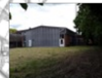
Old telephone exchange
